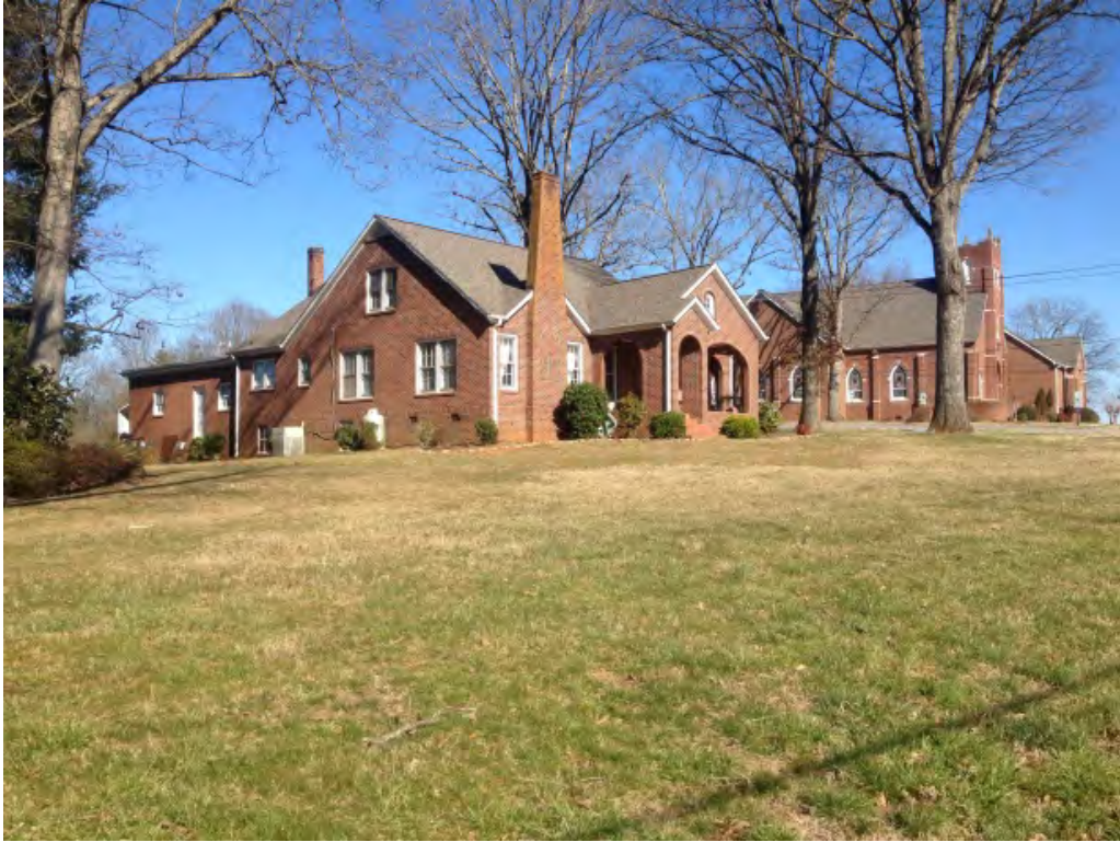
Oblique view of parsonage looking northeast
