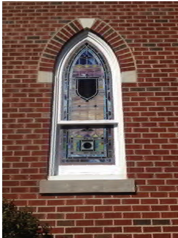
Lancet-arched windows with stained glass and wood frame
