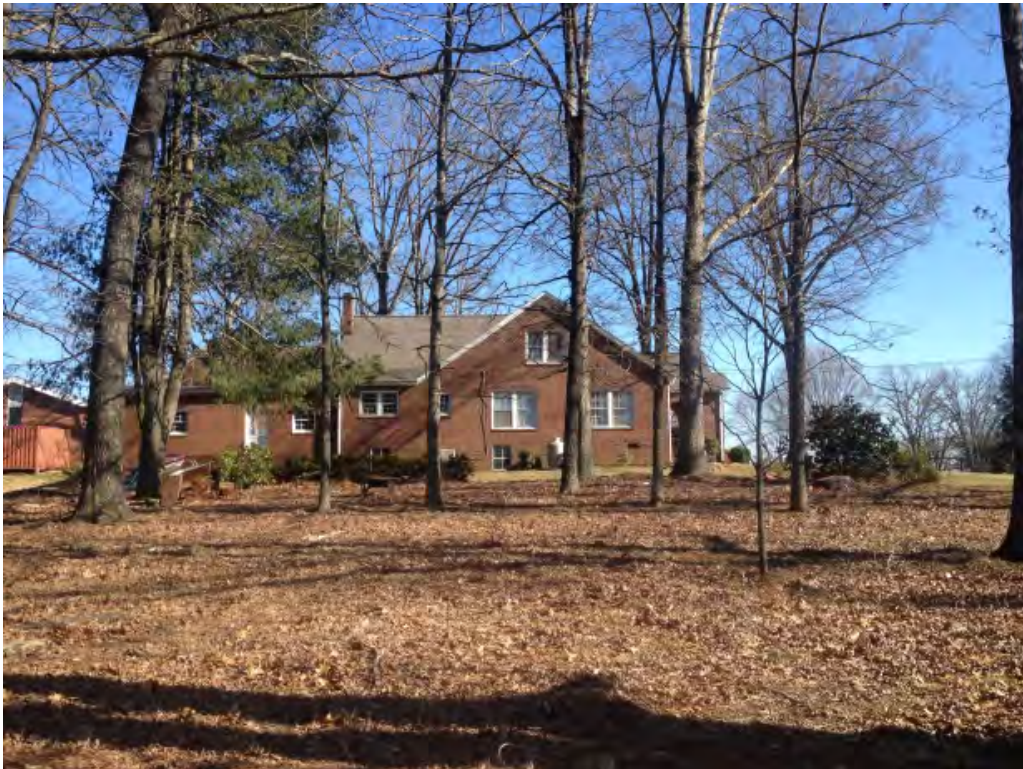
West elevation of parsonage
