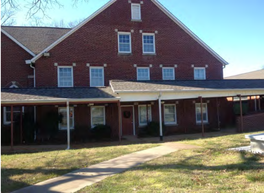
New Jerusalem Lutheran Church, 1948 educational building east elevation and covered walkway looking northwest
