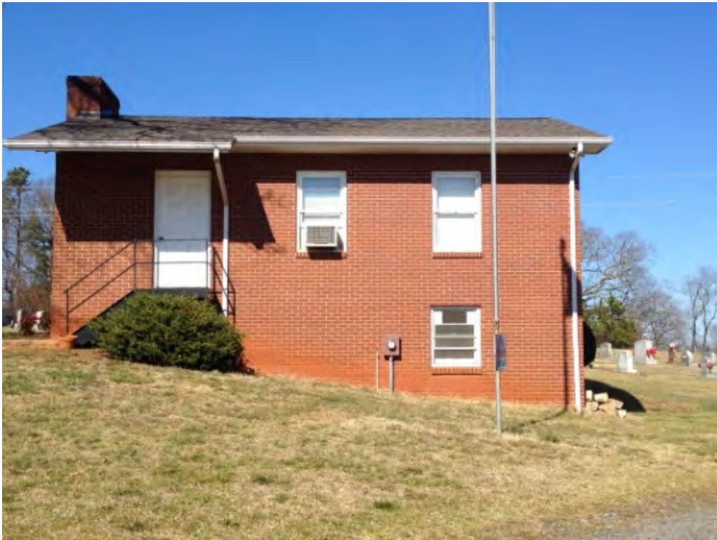
Boy Scout Hut façade looking north
