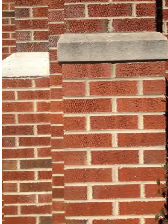
Concrete caps on buttresses
