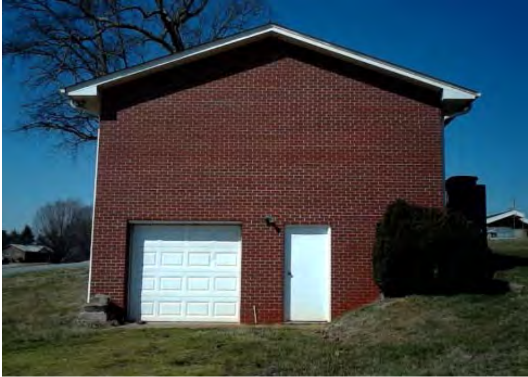
Boy Scout hut east elevation looking west
