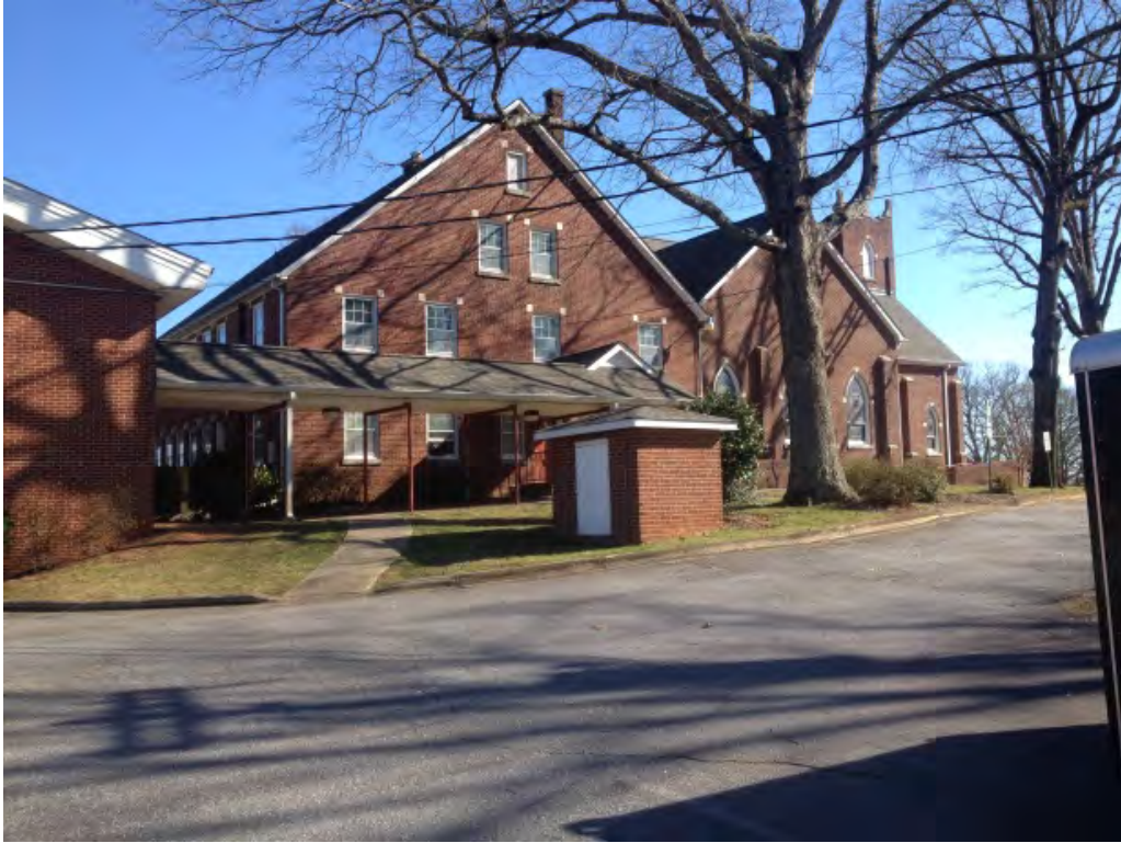
New Jerusalem Lutheran Church, west elevation looking southeast
