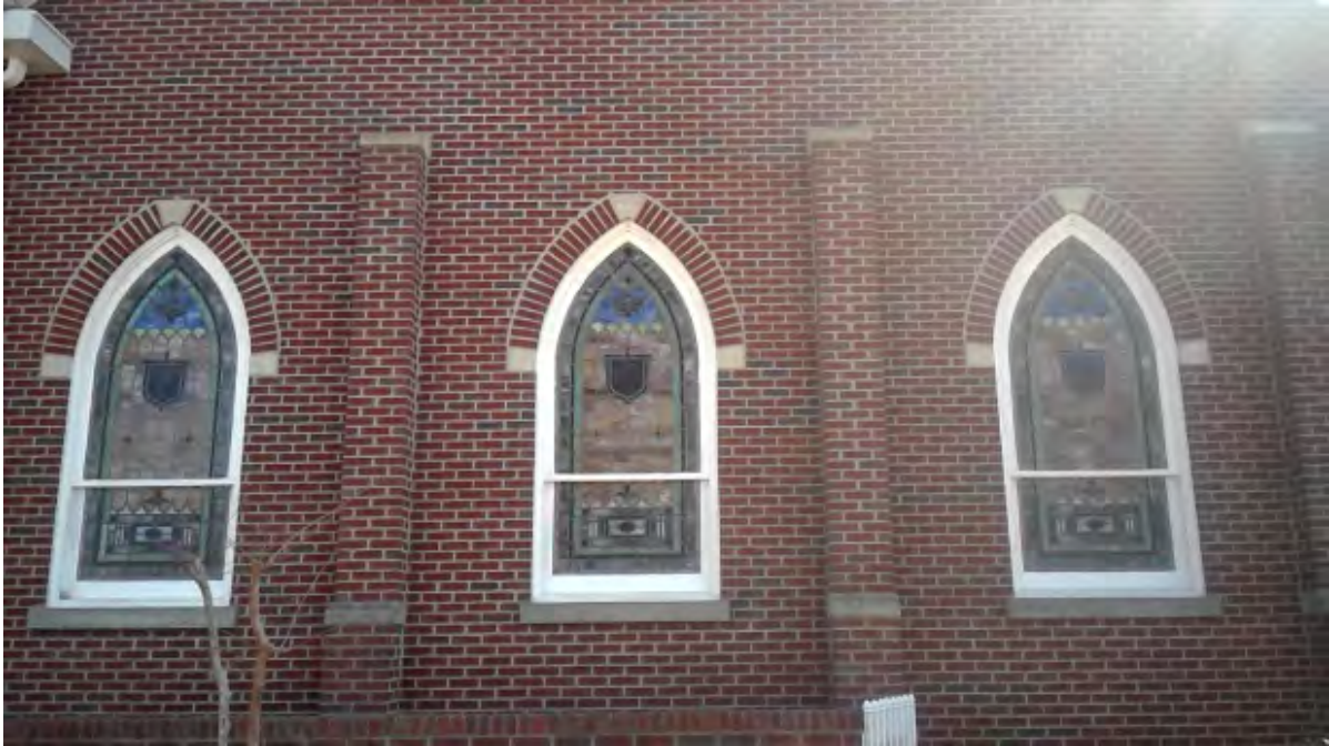
Buttressing between windows on 1948 building
