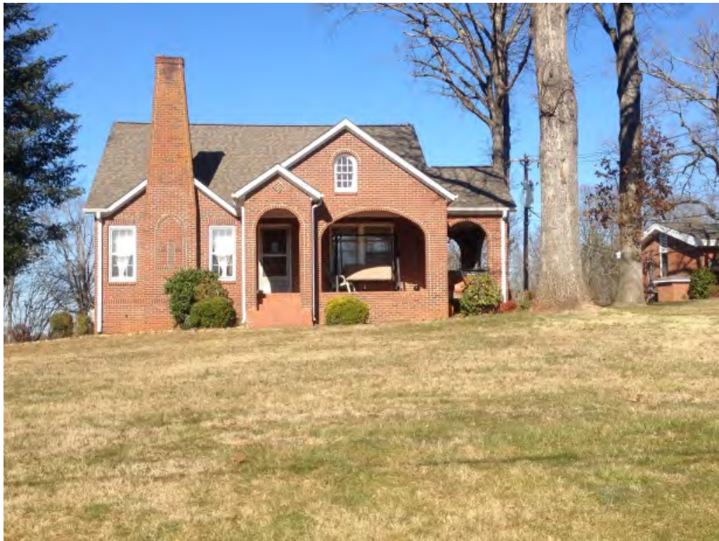
Façade of parsonage looking north
