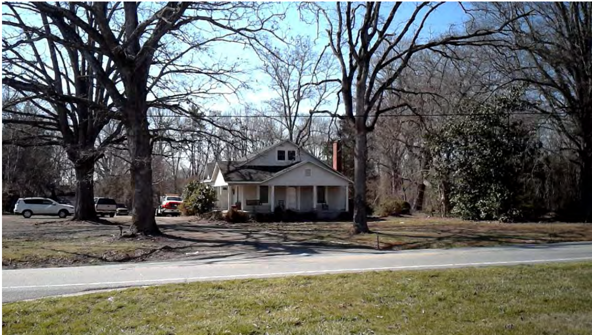
Old Killian School House now a residence located across Startown Road from church
