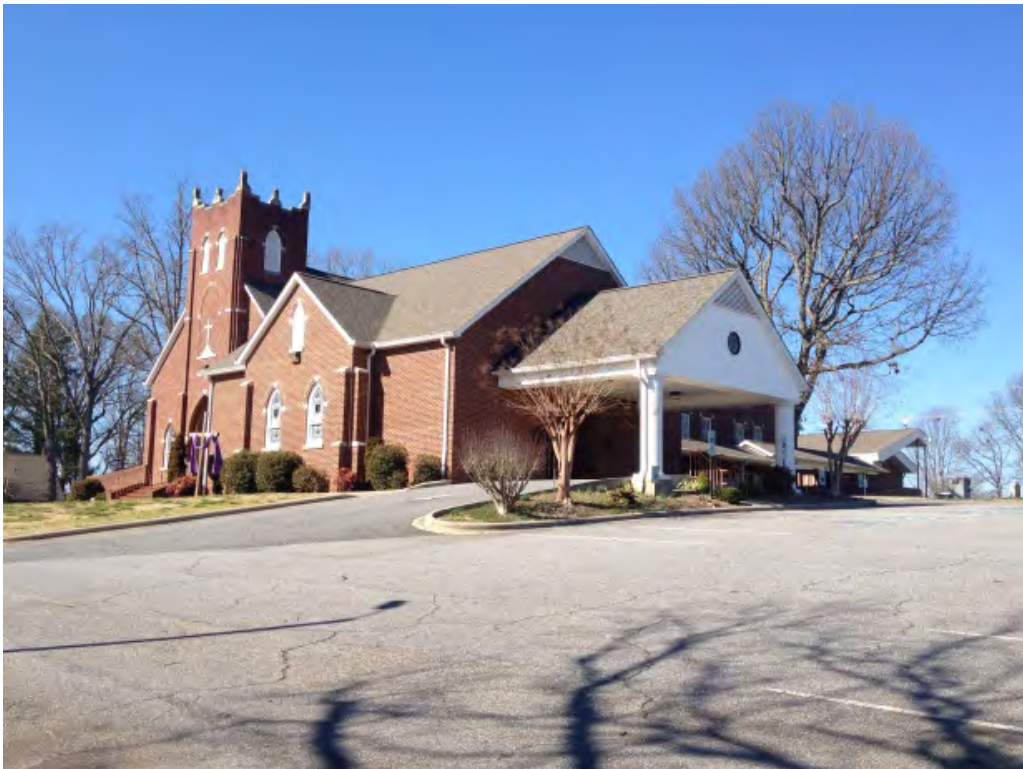
New Jerusalem Lutheran Church, 2001 addition with porte cochere looking northwest
