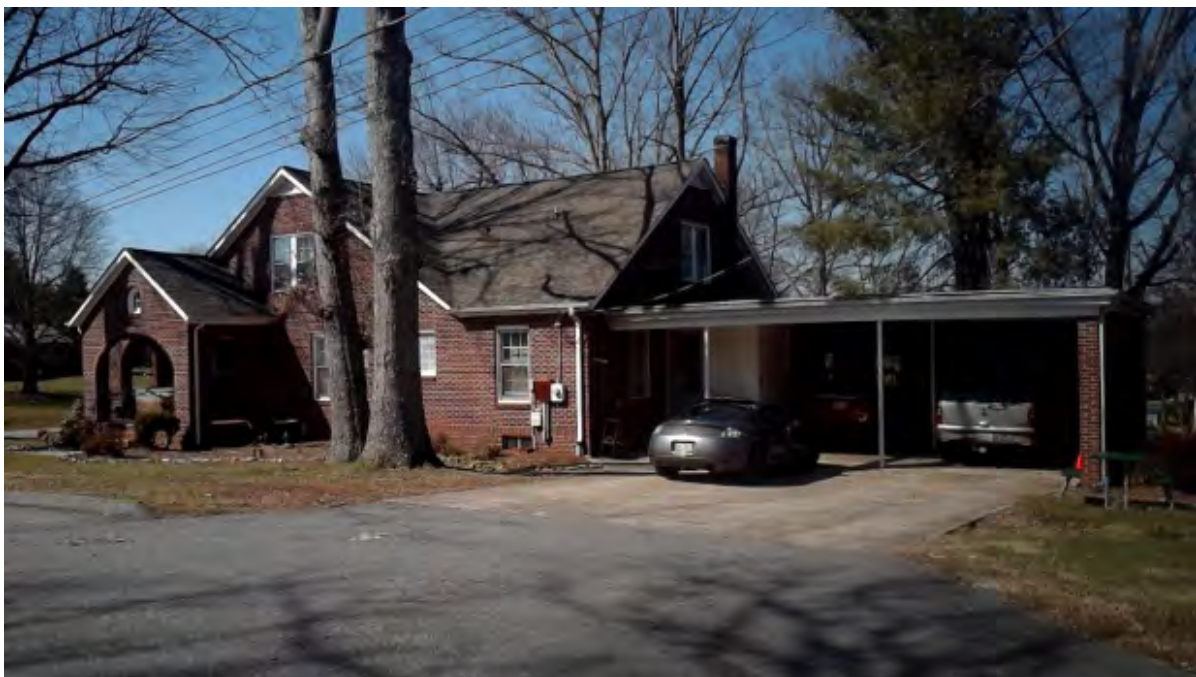
Oblique view of parsonage carport addition looking west
