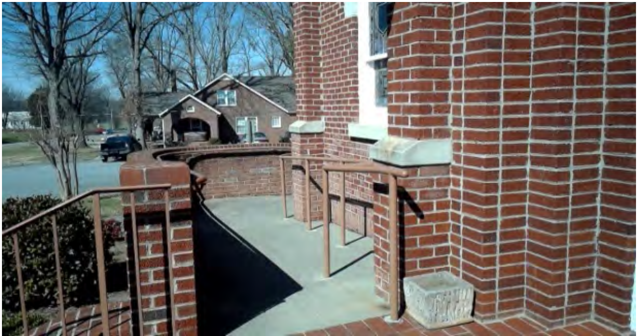
1984 ramp addition at front entrance
